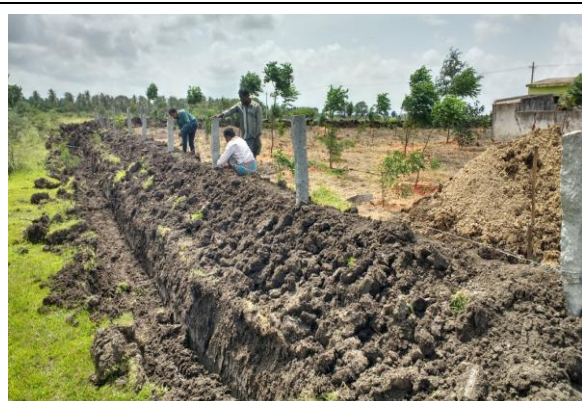
Fencing and rain water harvesting for soil and moisture conservation
